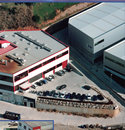
Arenys de Mar Plant
