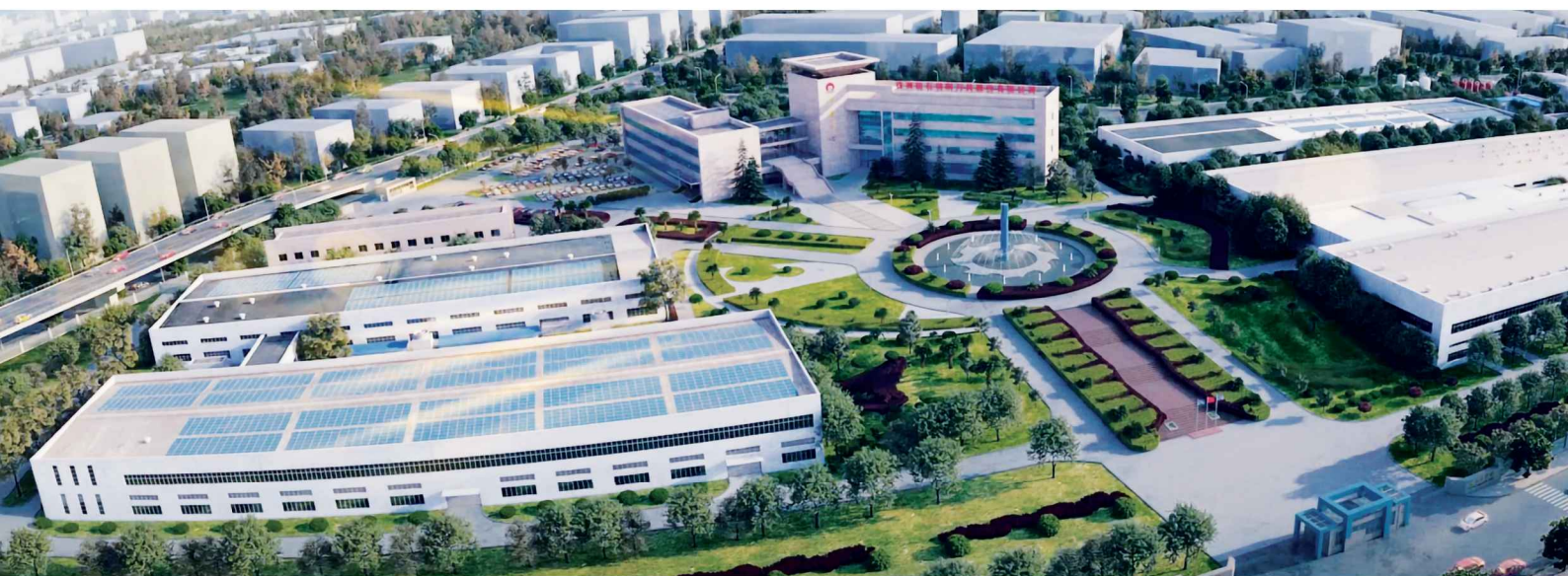
ZCC Cutting Tools Headquarters, Zhuzhou, China
